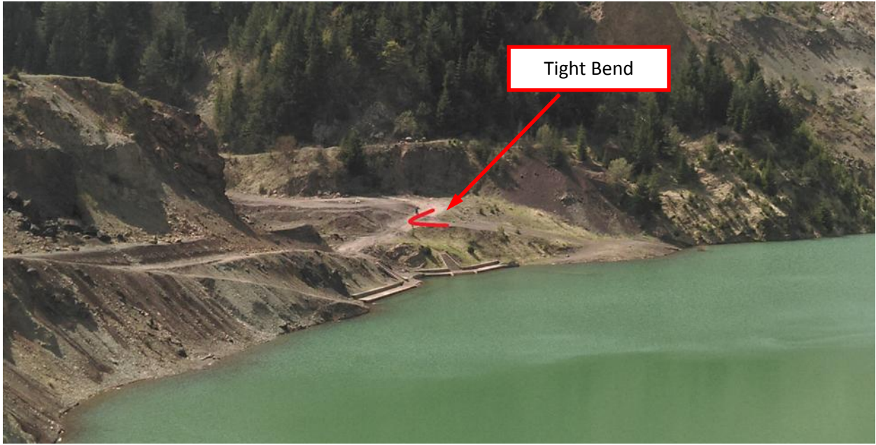
Figure 18 - 'South Beach' - indication tight bend
