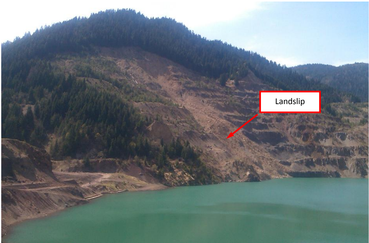
Figure 6 –Vares Mine – Landslip on south bank of open pit
