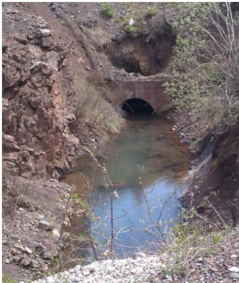
Figure 8 Vares Mine - Open tunnel section
