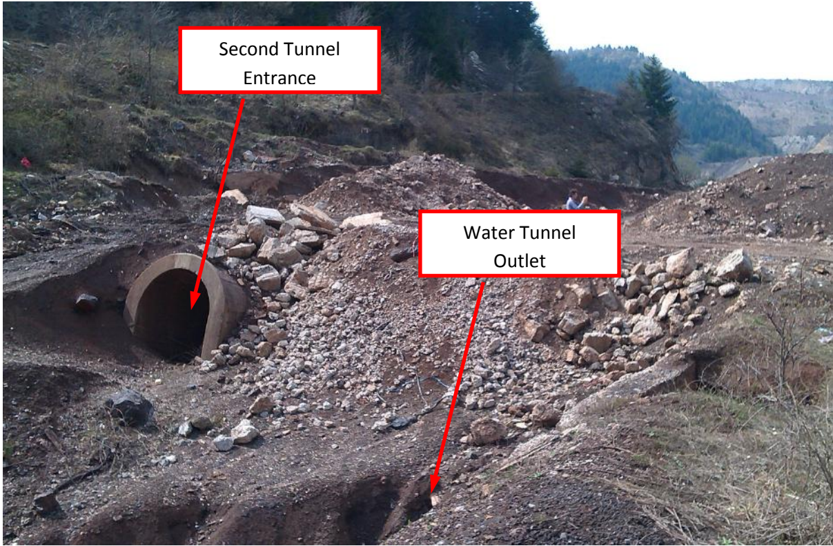
Figure 10 –Vares Mine – Tunnels to south of open pit
