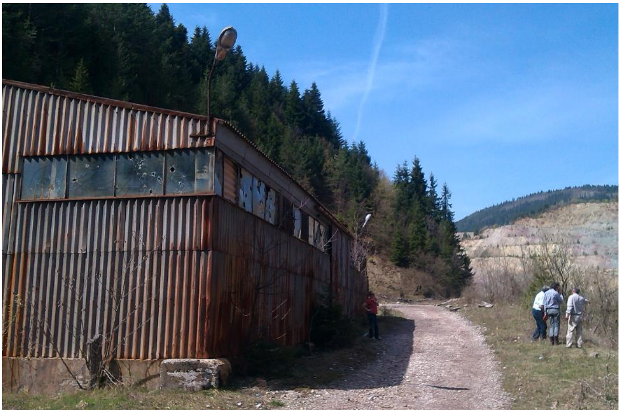
Figure 13 –Access to South bank of Vares mine looking North West in direction of open pit
