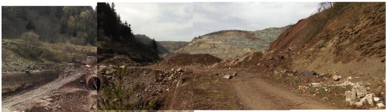
Figure 23 - Panorama proposed location for dewatering plant
